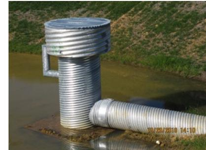
Perforated dewatering device attached to principal spillway.
