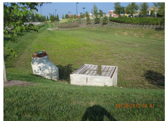
Figure 7. Landscaped and well-maintained permanent stormwater detention pond.
