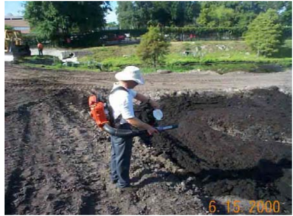
Figure 9. Application of flocculant powder to thicken bottom sediment slurry.
