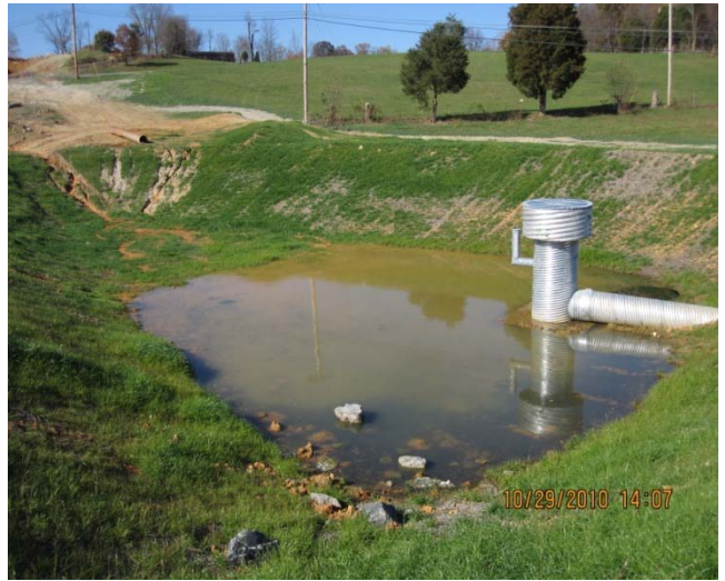
Figure 1. Typical sediment basin with dewatering device.
