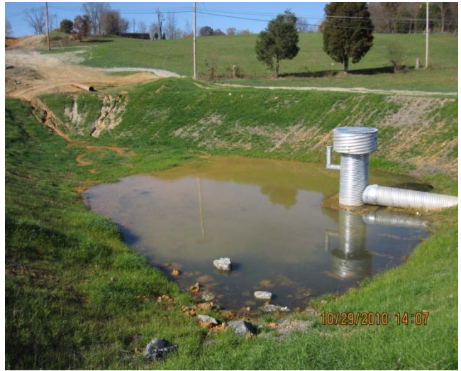
Figure 1. Typical sediment basin with dewatering device.
